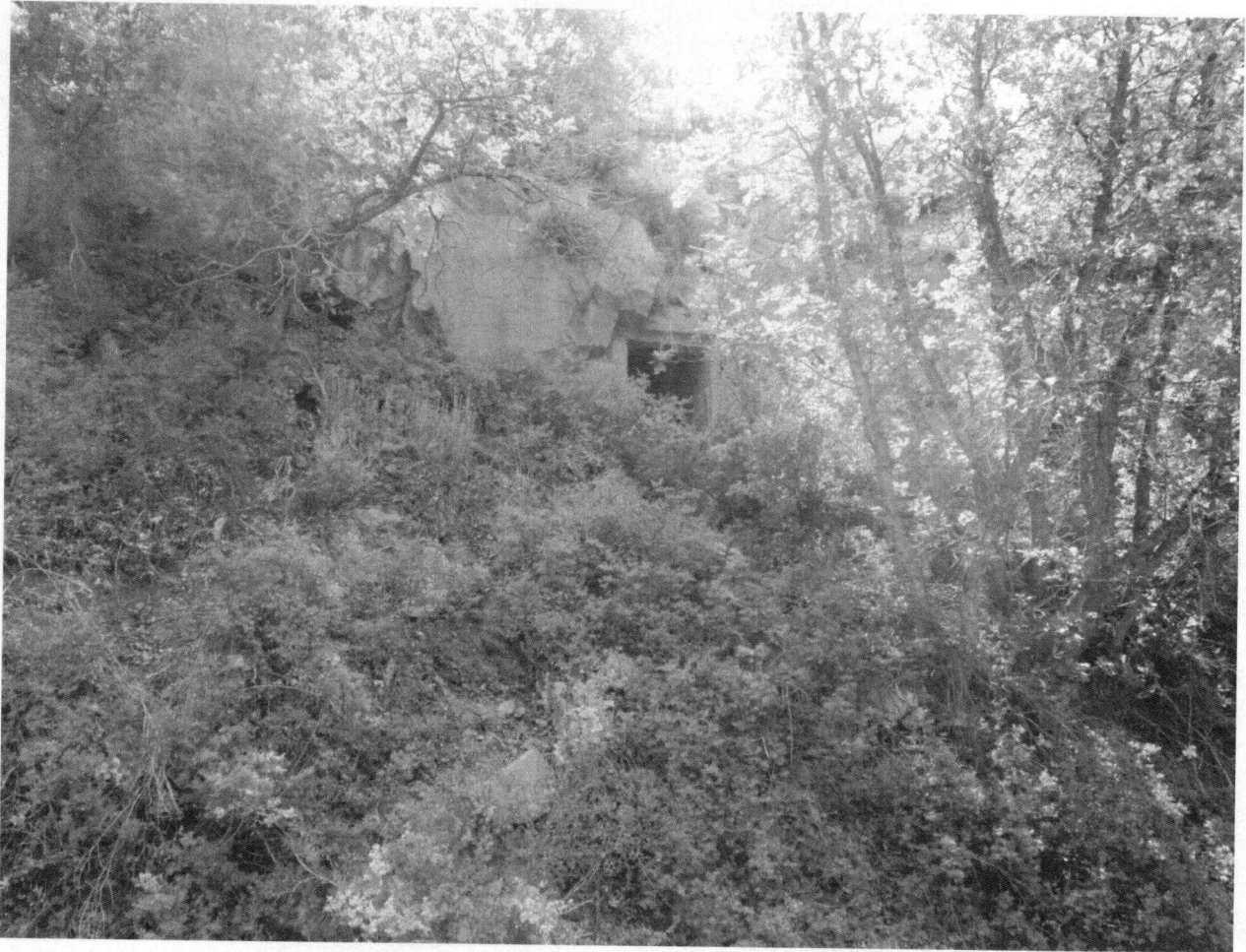
Photograph 50: Concrete structure likely associated with historical mining activities. Photopoint: KK UTM Coordinates: 503162 4396031 Bearing of Shot: 75 degrees
