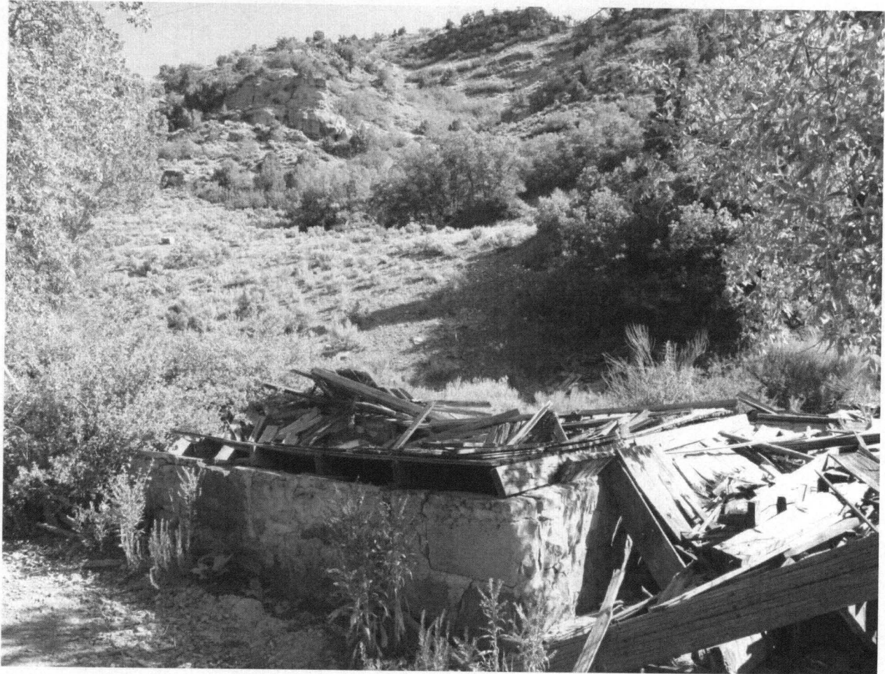
Photograph 31: Fallen historical structure. Photopoint: Y UTM Coordinates: 502840 4395823 Bearing of Shot: 5 degrees
