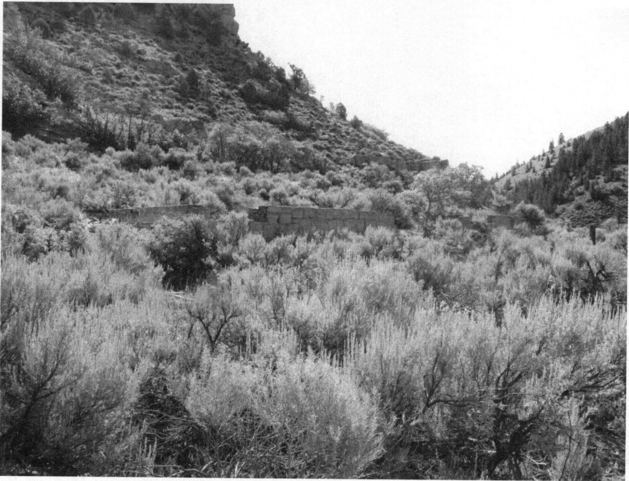
Photograph 46: Foundation of historical rock structure. Photopoint: HH UTM Coordinates: 503265 4395795 Bearing of Shot: 75 degrees
