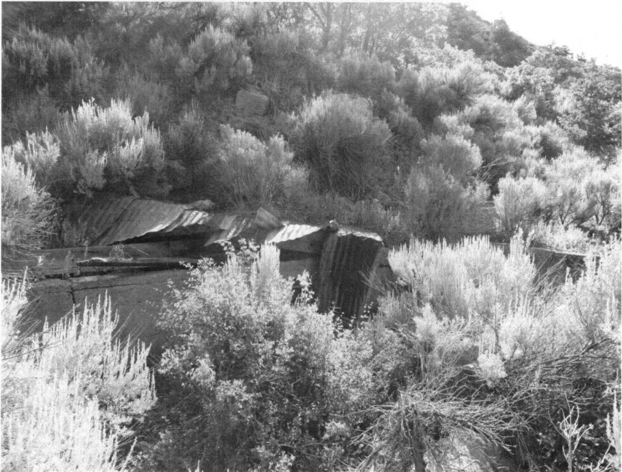
Photograph 23: Typical building foundation remaining from the ghost town Mutual.
