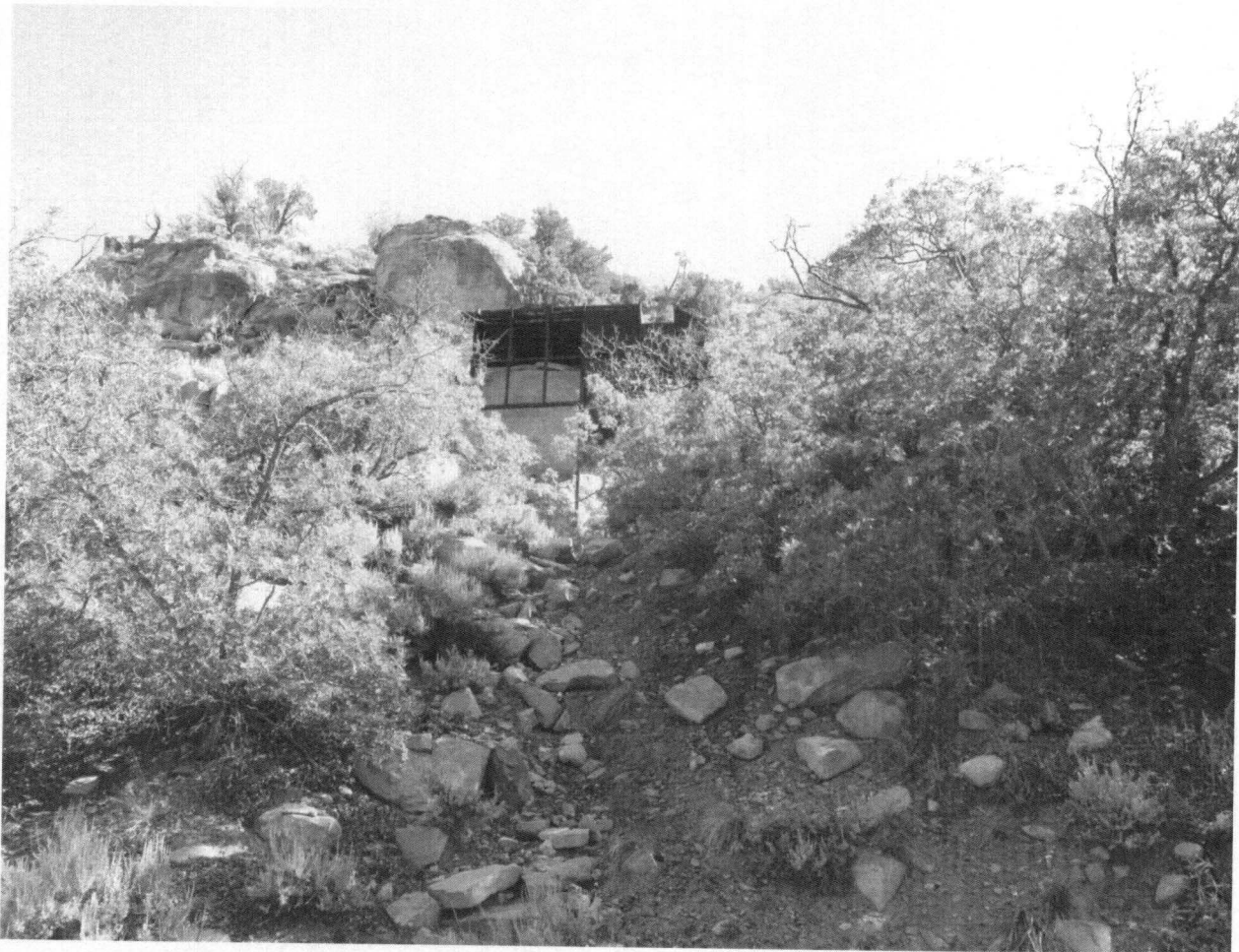
Photograph 34: Historical mining structure. Photopoint: BB UTM Coordinates: 503022 4395546 Bearing of Shot: 20 degrees
