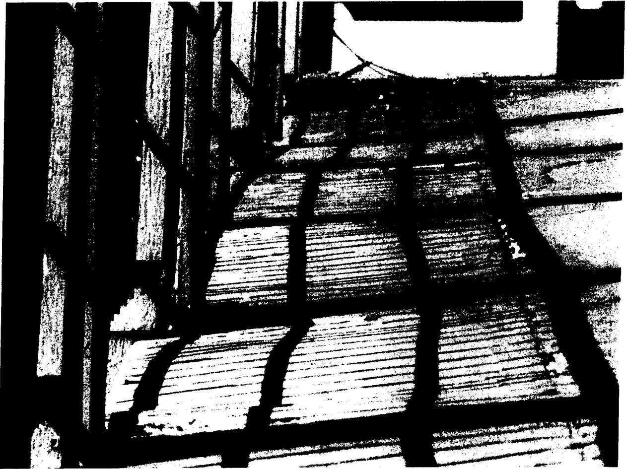
Picture 11: Multiple points of support for the balcony structure have failed and are failing.
