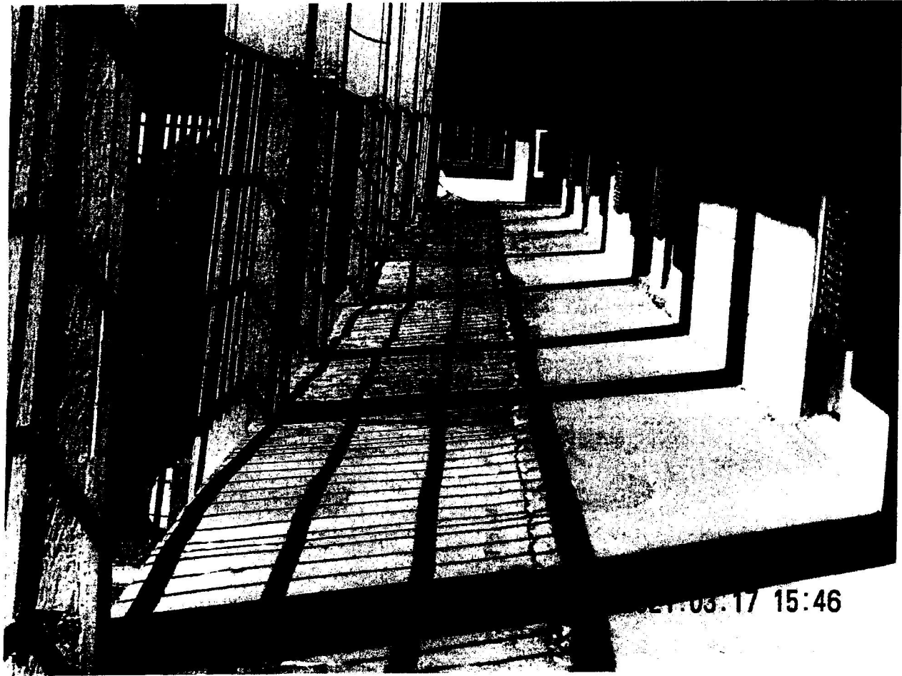
Picture 12: The upper balcony has failed to a point there is a large separation in elevation.
