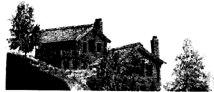
Construction on steep slopes should attempt to avoid cutting into existing topography for foundations.
