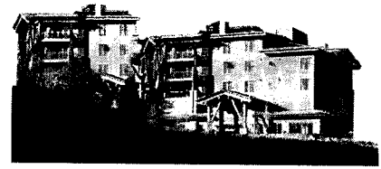
Buildings on natural topography above 15 percent in slope shall be stepped in form.
