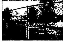
6' RUBBER-COATED CHAIN LINK FENCE
