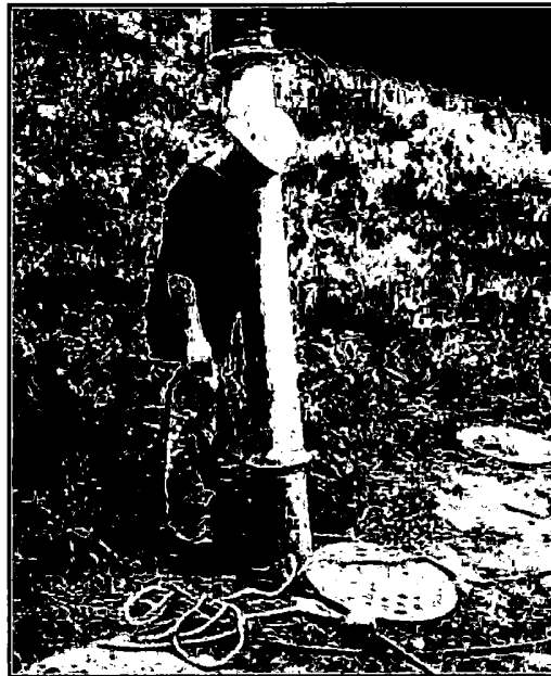
Vacuum (vactor) truck quickly cleans the single open access swirl chamber
