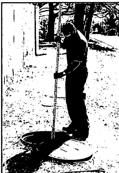
Sediment inspection using a stadia rod
