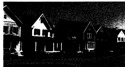
Not this - Similar two-story homes repeated too often
