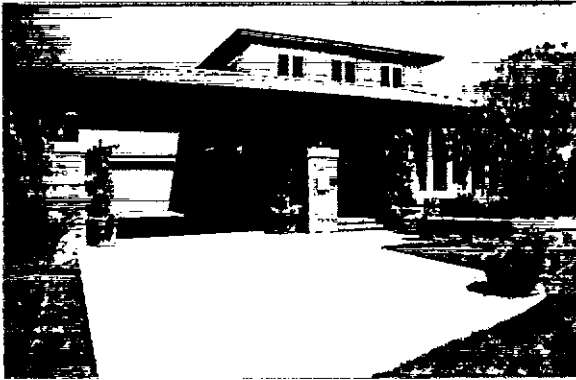
Porte cochere and oversized brick columns
