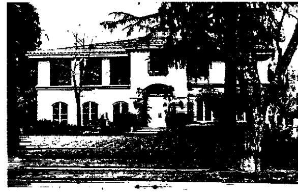
Belt course trim and arched windows
