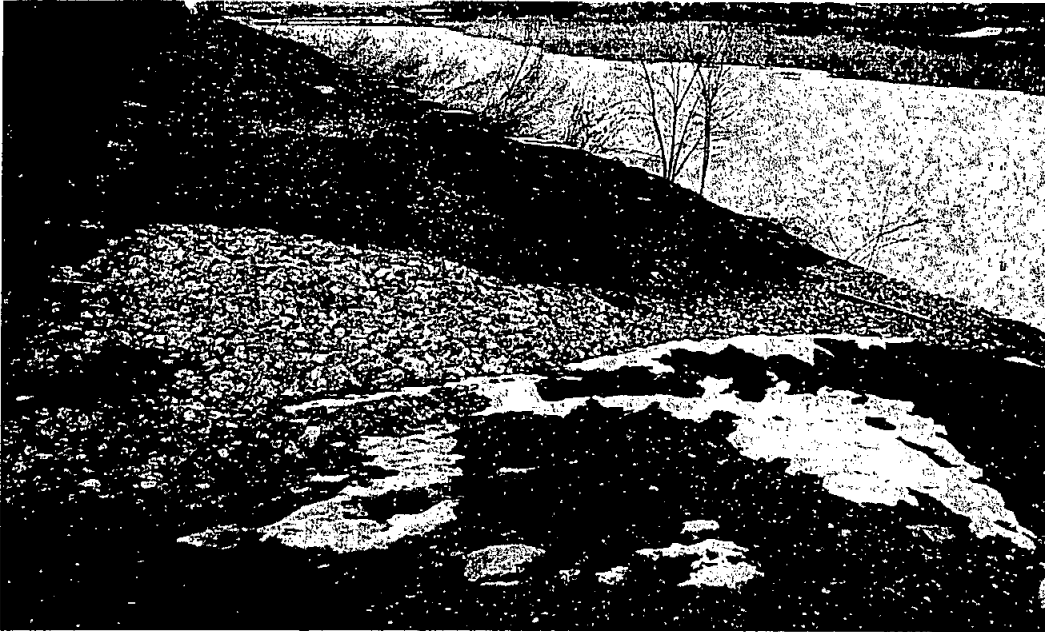
Photograph 7: A look at a rock drain that starts on the freeway side of the fence and flows east into pond 4. There are approximately 3 entering pond 4 and 1 entering pond 3. Photopoint: G
