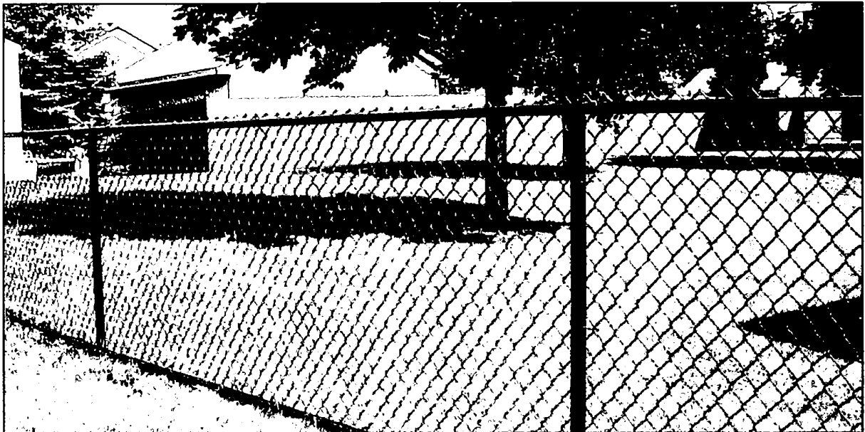
Canal Fence (adjacent to canal): 6' black or dark green vinyl coated chain link
